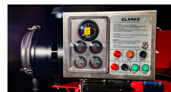
NEMA 4X/IP66 Stainless Steel Instrument Panel
