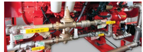
Sea Water Cooling Loop
